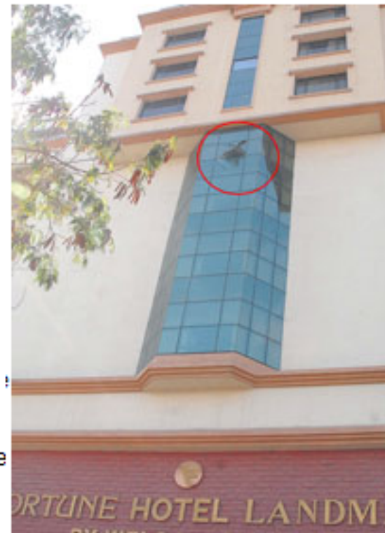
HANGING ON: A worker (circled) seconds after he dashed against a glass panel on the hotel's fifth floor on Sunday
